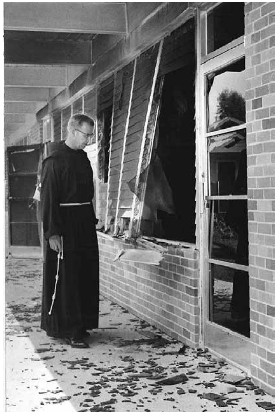
Christopher Schneider, OFM, surveying the damage to Our Lady of Good Harbor School, Buras, Louisiana, August 28, 1963. The school would not be reopened (Courtesy of the Associated Press).
